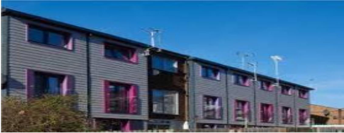
Photo Energiesprong retrofit homes pilot Sneinton
