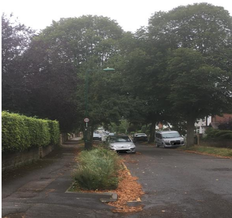
Photo of Rain Garden Ribblesdale Road, Nottingham
